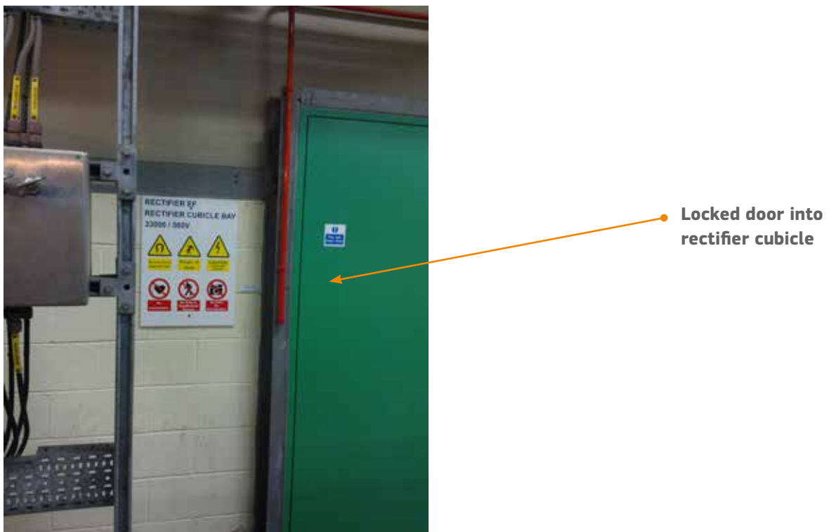
Figure 3.3 — Restriction of access to a rectifier cubicle bay
